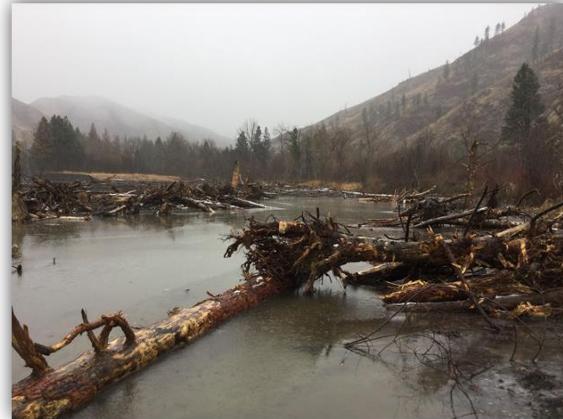
Figure 18: The upper left image was taken in March 2019 and illustrates the upstream extent of the Rainbow Lake dam removal that took place in 2018 as part of the WDFW lead Floodplain Management Plan. The yellow arrow indicates the previous position of the dam/levee that was removed. Following the removal of the dam the area that was previously lake bed was roughened with LWD and will be planted with wetland plants in the spring 2019. A flow path was developed through the previously inundated area (upper right) however this area remains disconnected from the river by levees which will be addressed during the implantation of PA13 in 2020. The lower right image shows the downstream end of the treated area.
