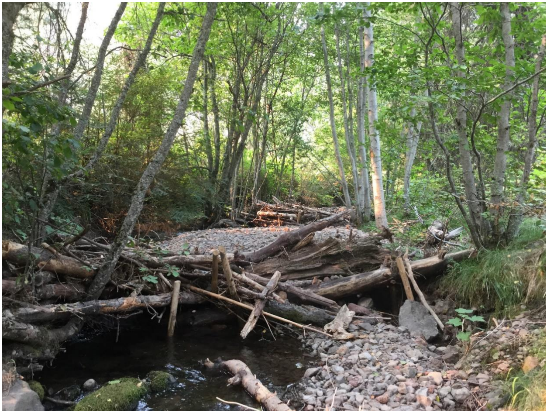
Figure 27: In 2018, the CCD conducted a Post Assisted Log Structure project on the Little Tucannon River for the purpose of generating bed load and storing it. The upper image is a post project photo before high flow and the lower image is a structure following flow and grave deposition around the structure.
