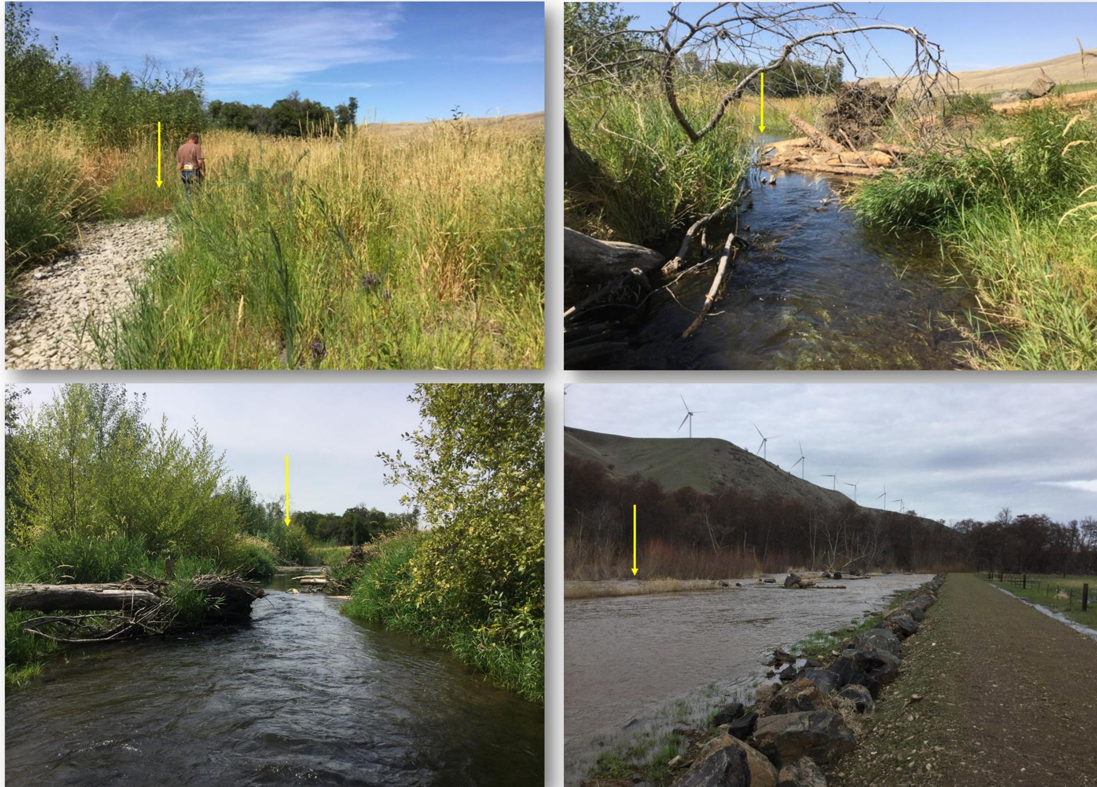
Figure 21: Phase I side channel pre project (upper left) immediate post project (upper right) and post high flow 2017 (lower left). The lower left photo shows the level of the flow in March 2017 and ~1,100 cfs. Flows during the flood extended across the entire floodplain and exhibited relatively shallow depth and low velocities. Flowing the flood very little scour was observed on the floodplain, however some areas had >2" of fine sediment deposition and residual pools depths within the channel exceed 1.5 m in some areas. The yellow arrow indicates the same general location through the time series.
